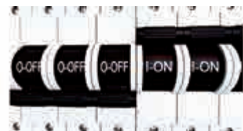
Figure 2.23 Set of trip switches
